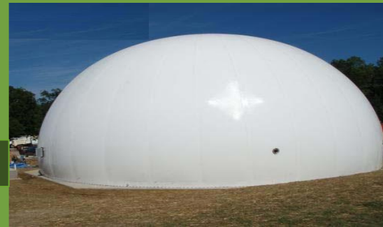
Purified Gas Storage Balloon
